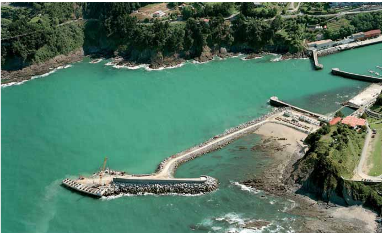
Construction of wave energy plant, Mutriku, Spain
